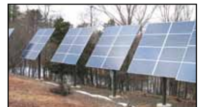
Solar panels at Lifebridge Sanctuary in Rosendale Photo by Patty Matteson
