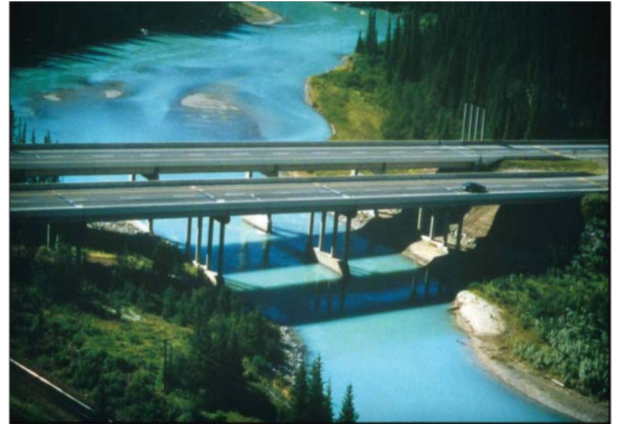
Figure 40. Photo. Wide span viaduct designed to conserve floodplain (Credit: Tony Clevenger).
