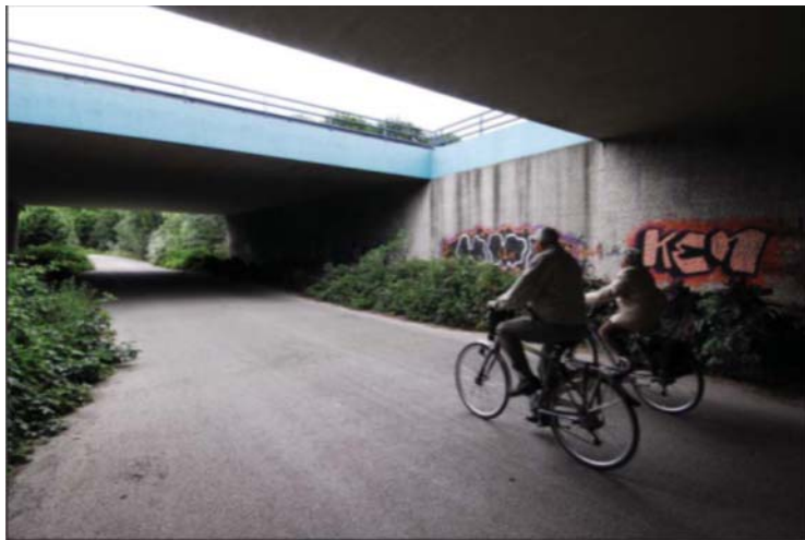
5. Photo. Multi-use underpass in The Netherlands retrofitted for human use and wildlife passage (Credit: Marcel Huijser).
