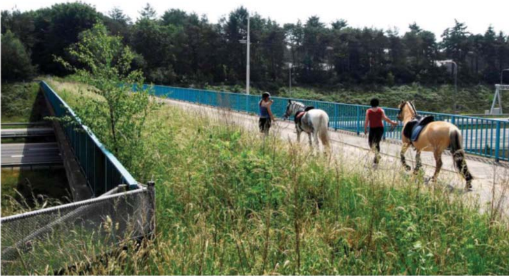
Figure 36. Photo. Human use lane and vegetated strip on multi-use overpass (Credit: Marcel Huijser).
